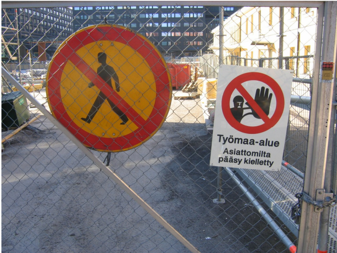
Fig. 1. View at a construction site
